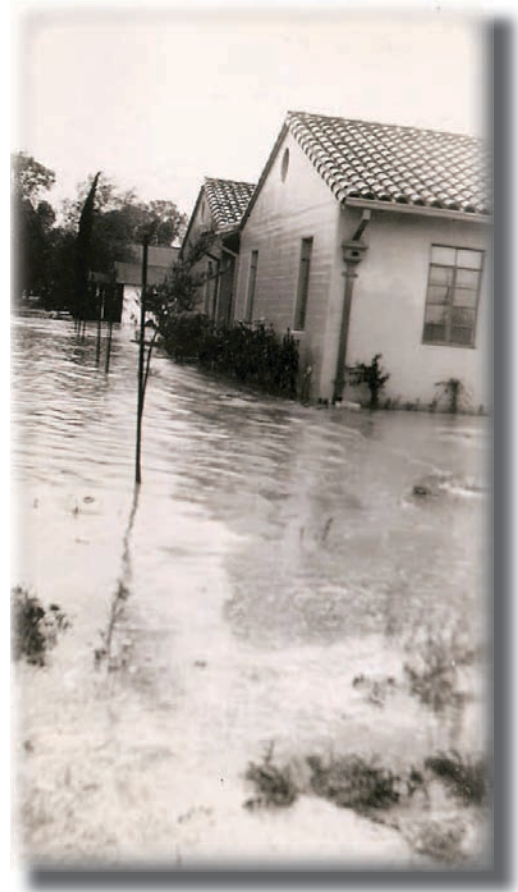
Right; Looking west to the rear of Station 1 after the flood waters settled.
