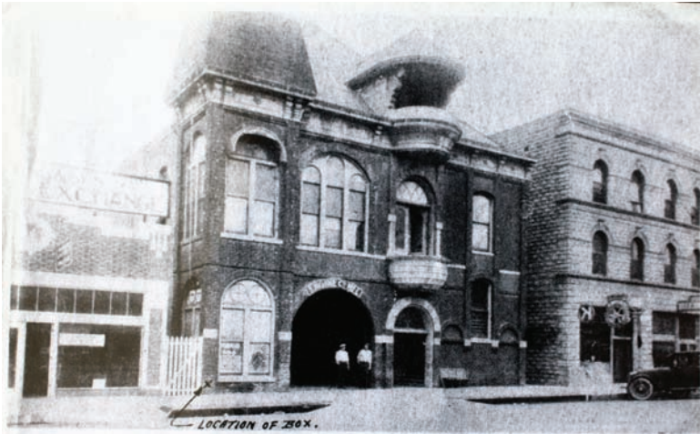
THE CITY HALL OF COLTON as it appeared in 1924, prior to major remodeling and strengthening of the 1890 structure. The building was demolished in 1965 and the contents of a cornerstone, indicated by X, was found in a salvage yard by a Rubidoux man. The contents of the box were returned the city last week as the first donation for the city's proposed museum.
